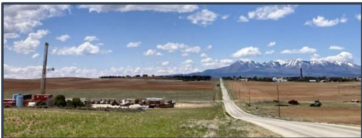
Figure 1 – Aztec 980 Drill Rig on Jesse#1A well site in SE Utah
