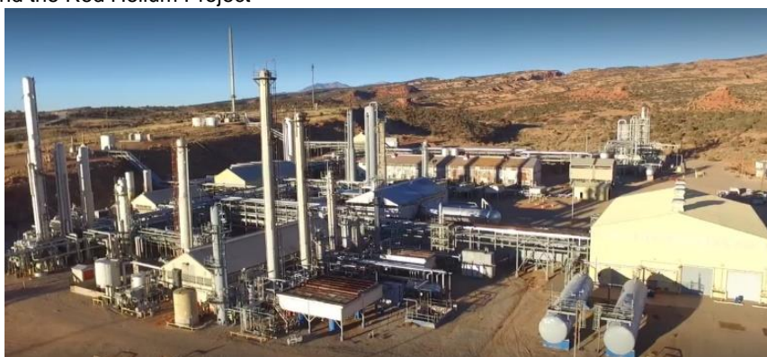
Paradox Resources “5 1/2 Nines” Lisbon Valley Gas Processing Plant.
