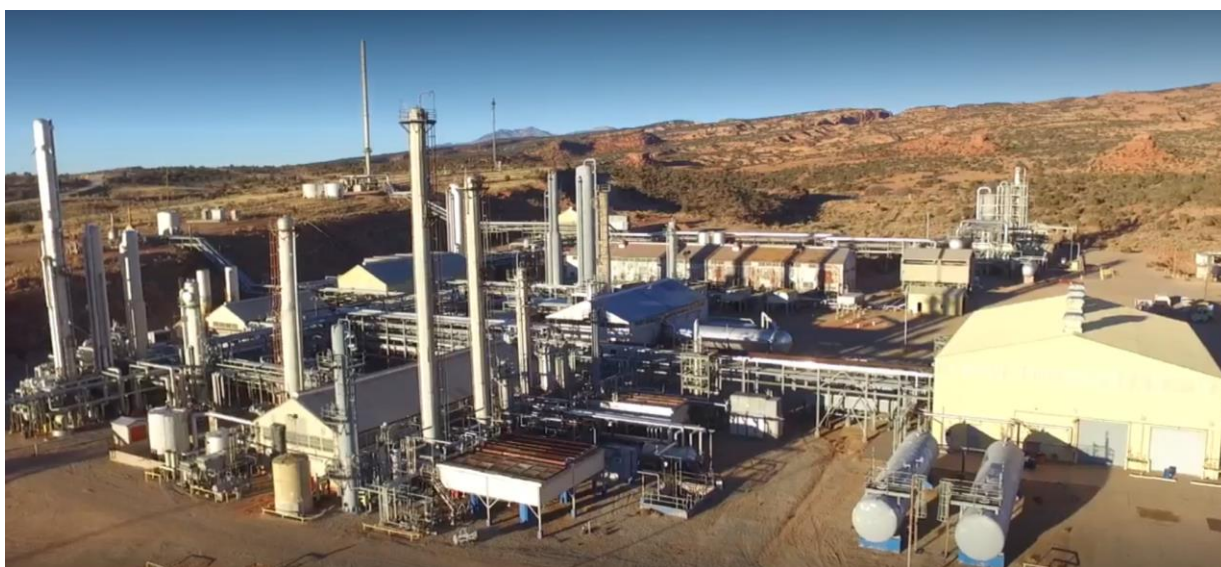
Figure 2: Paradox “5.5 Nines” Resources Lisbon Valley Gas Processing Plant.
