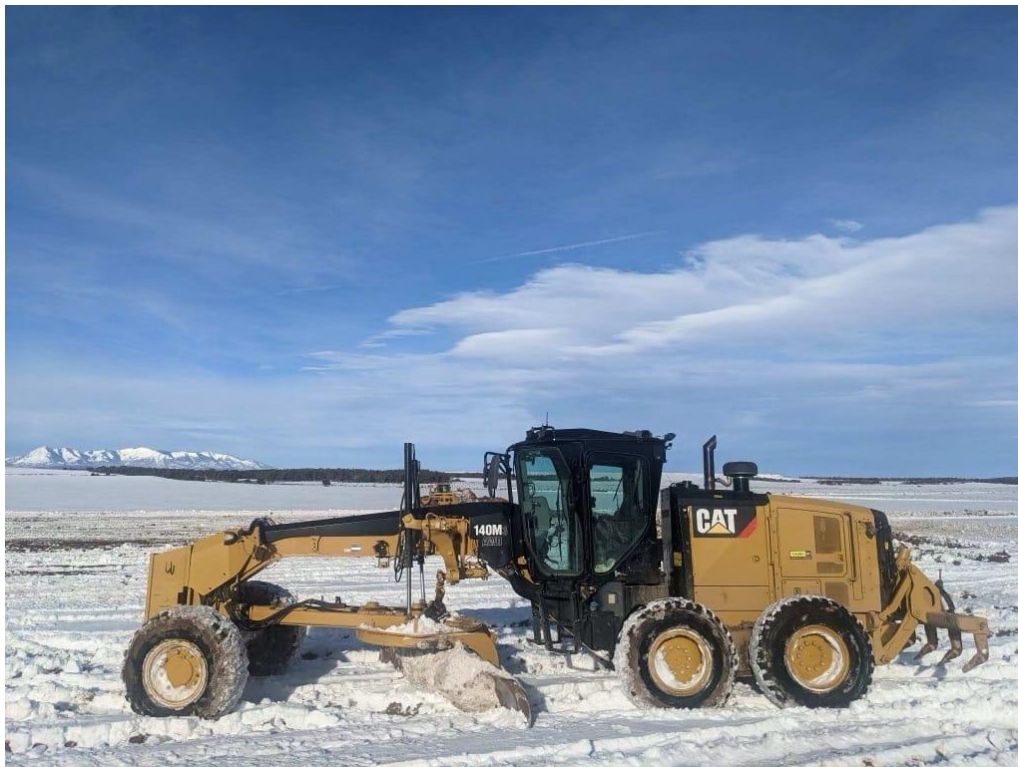
Figure 2: Jesse-2 well pad construction begins in Utah
