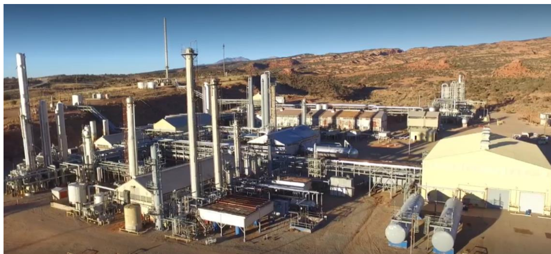
Figure 4: Paradox “5.5 Nines” Resources Lisbon Valley Gas Processing Plant.
