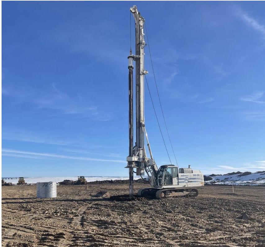
Figure 1: Conductor rig on the Jesse-2 well site in SE Utah.
