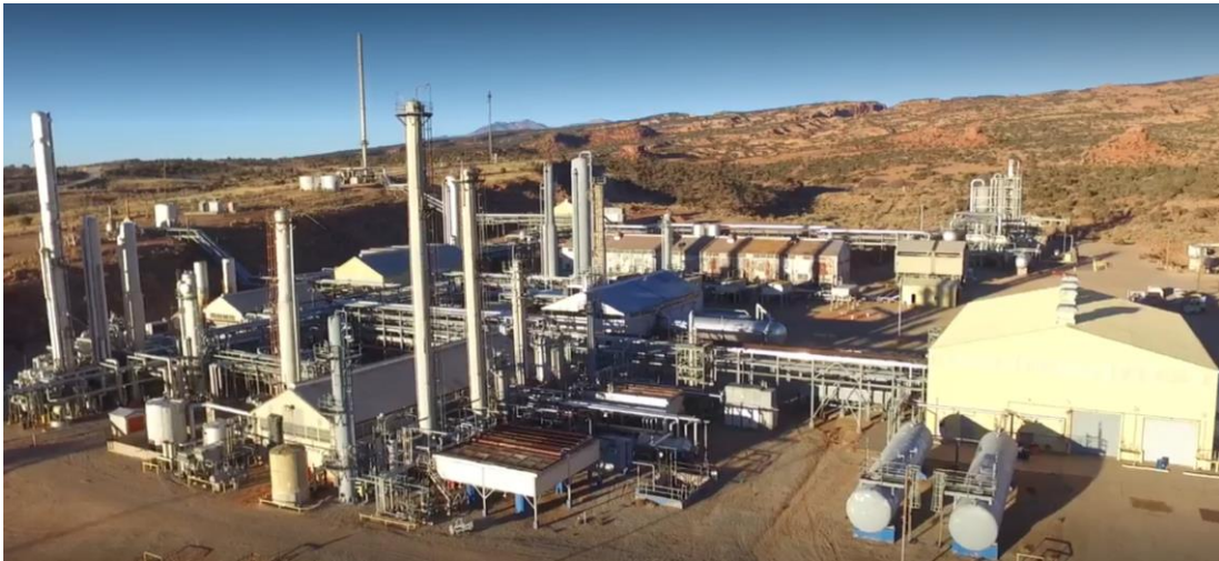
Figure 5: Paradox “5.5 Nines” Resources Lisbon Valley Gas Processing Plant.
