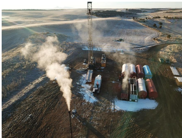
Figure 2: Jesse-1A well-site with flare-stack venting reservoir gas and helium to surface during flow-testing
