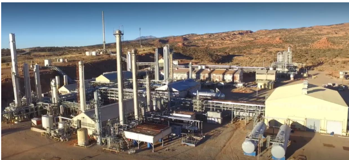
Figure 2: GNG Advanced Lisbon Valley Helium Processing Plant
