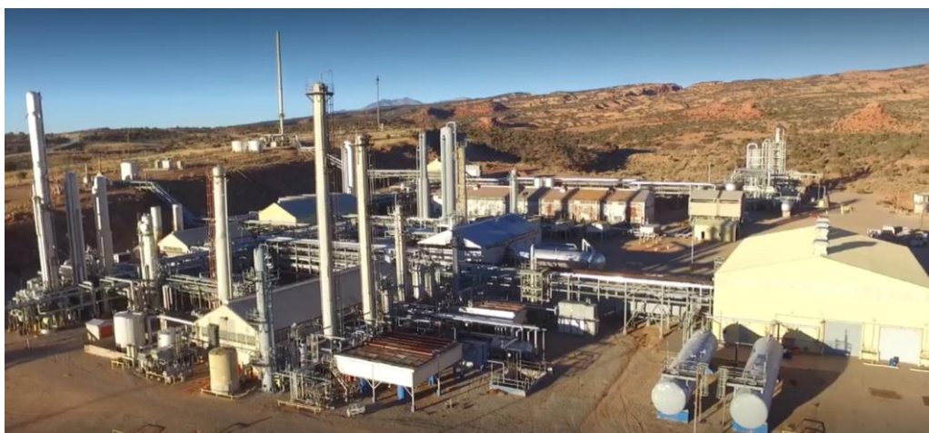
Figure 2: "5.5 Nines" Advanced Lisbon Valley Gas Processing Plant.
