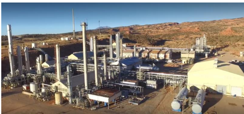
Figure 2: "5.5 Nines" Advanced Lisbon Valley Gas Processing Plant.
