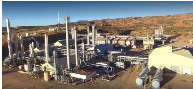
Figure 3: "5 1/2 Nines" Advanced Lisbon Valley Gas Processing Plant.
